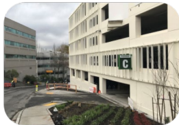
Fall 2018 Parking Garage C Construction Completed
